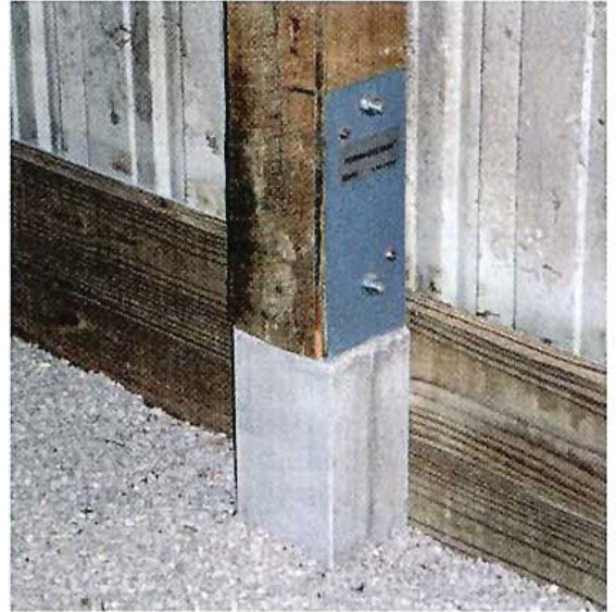
LEFT: This rotted post was just 20 years old. RIGHT: The Perma-Column replacement keeps wood from contacting soil.
